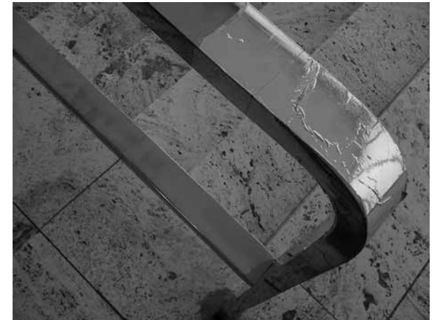
Image: Villa Tugendhat, one week before restoration Photography by architecten de vylder vinck taillieu
