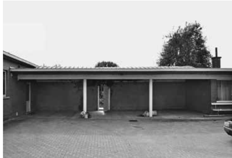
Image: Original situation Photograph by Wim Goes Architectuur
